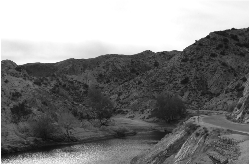
Little Rock Dam
