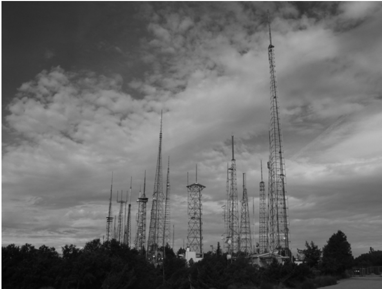
Mt. Wilson Telecommunications Site
