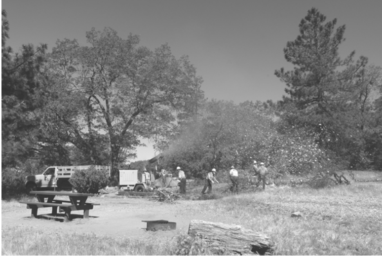
Arrowhead North Shore Campground—dead tree removal
