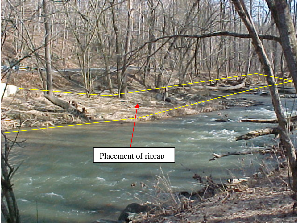
View showing approximate area of placement of riprap east of the bridge over Seneca Creek.
