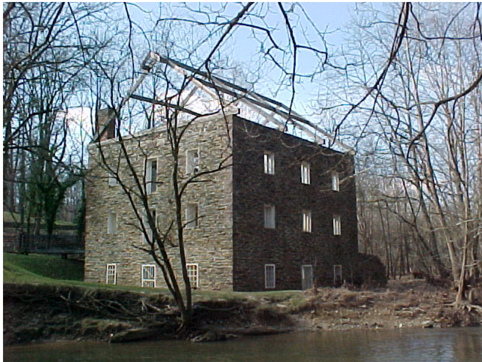
View showing Blackrock Mill looking west.
