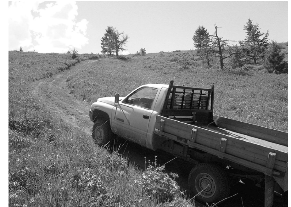
An example of a road with erosion potential due to steep grade
