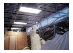
Cleaning the mold also does not fix the underlying moisture problem that is allowing the mold to grow. Mold should not grow without a moisture source, so if mold is growing on a wall, there may be a hidden leak somewhere or there may be a problem with water intrusion from outside. If mold is growing on sheet rock, there are may be a larger, hidden problem inside the wall space, which is not accessible without removing the sheet rock.
