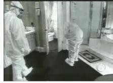
Thus, when conducting mold abatement with *Stachybotrys*, it is necessary to fully remove all of the airborne spores as well as the physical growth from the building. This requires additional air filtering and air exchanges during abatement.
