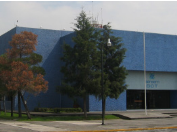
Building Housing WRS in Mexico City, Mexico
