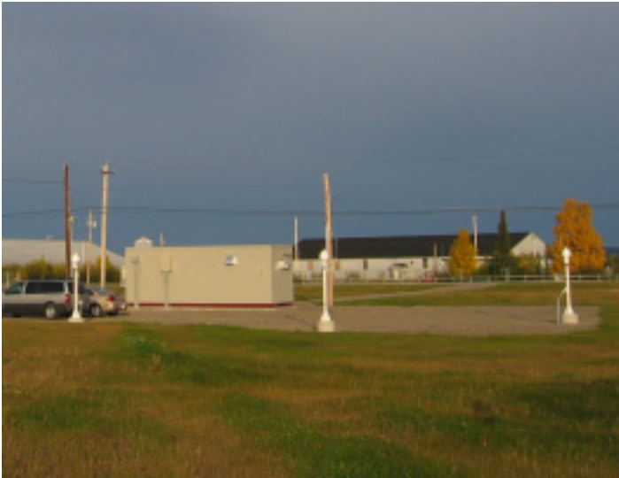
Building Housing WRS in Goose Bay, Canada
