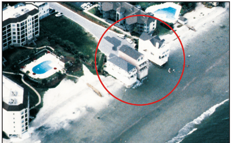
Figure 1. Well-built but poorly sited building.
