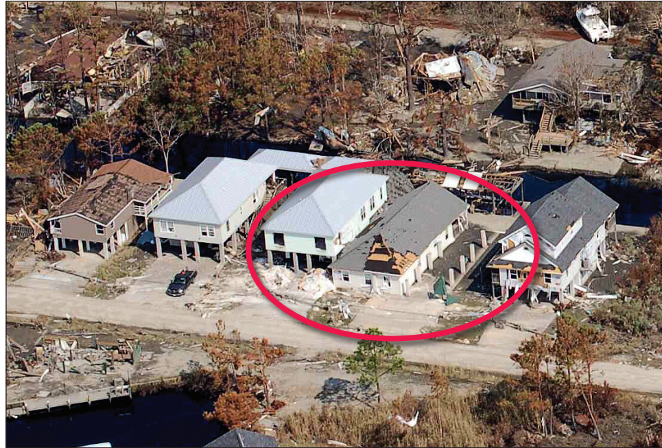
Figure 1. Damage to residential properties as a result of Hurricane Katrina's winds and storm surge. Note the building that was knocked off its foundation (circled).
