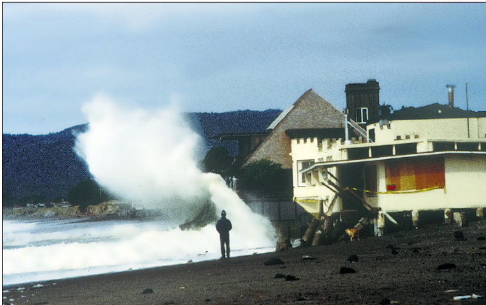
Figure 1-10. Storm waves breaking against a seawall in front of a coastal residence at Stinson Beach, California
