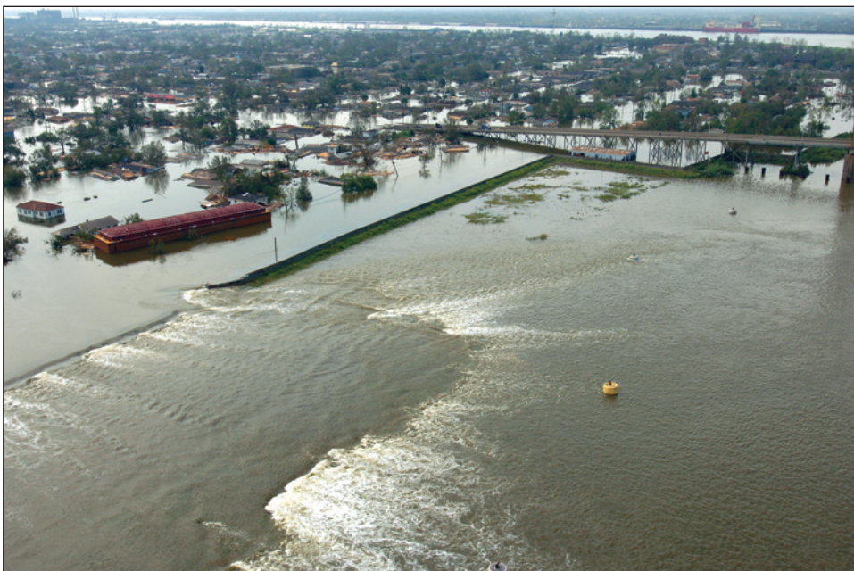
Figure 1-8. Aerial view of damage to one of the levees caused by Hurricane Katrina (photo taken on August 30, 2005, the day after the storm hit, New Orleans, Louisiana).
