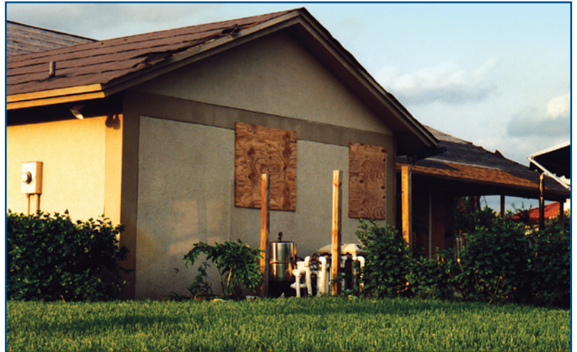
Plywood panels are a cost-effective means of protection.
