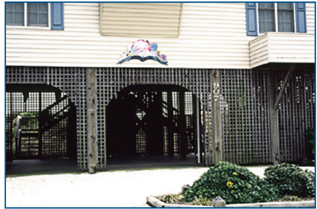
Open wood lattice installed beneath an elevated house in a V zone.
