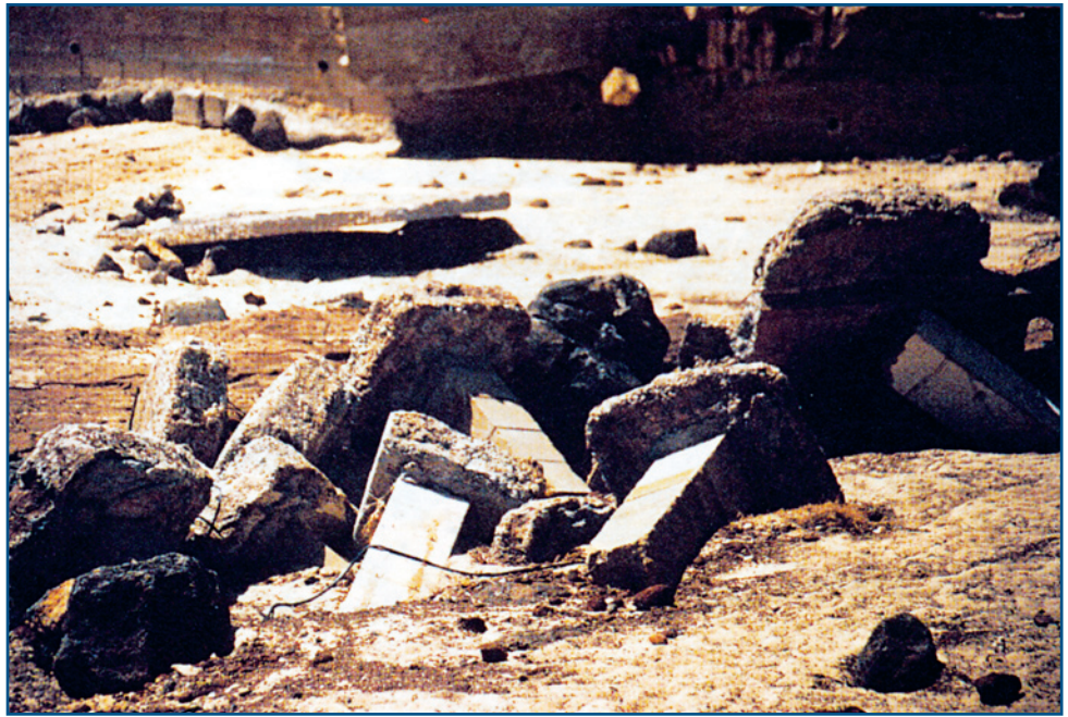
The small footings on the piers in this photograph did not prevent these piers from overturning during Hurricane Iniki.
