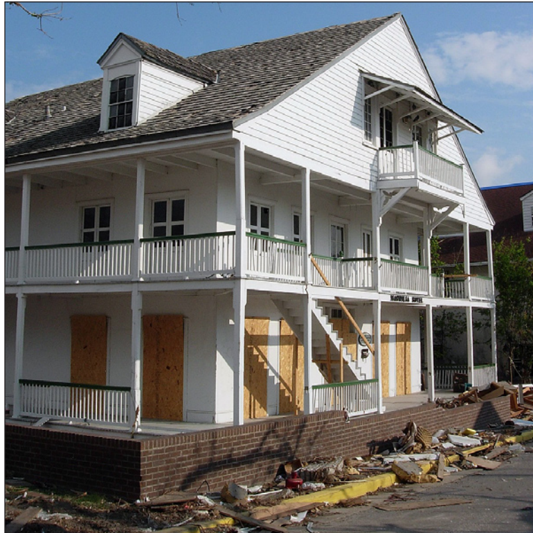
Figure J-1. Built by John Holm in 1847, the Magnolia Hotel, badly damaged from Hurricane Camille in 1969, was moved 100 yards north and restored by the City of Biloxi in 1972. While the main structure remains intact, the wood railing and one wood stair to the second floor porch were damaged; the other wood stair was completely destroyed (Biloxi, Mississippi).
