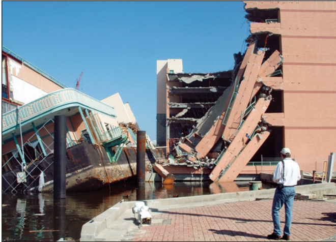
Figure 2-10. Parking deck collapse due to impact by casino barge, on left (Biloxi, Mississippi)
