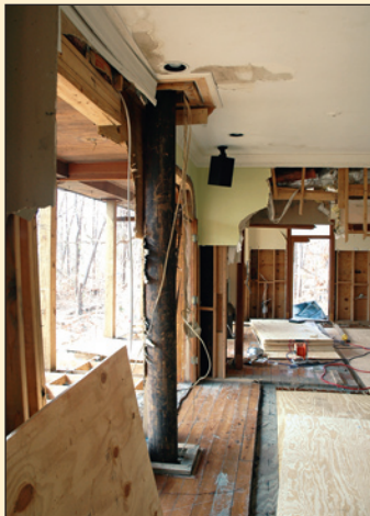
Wave damage to floors and walls, but pole construction left a repairable, surviving building.
