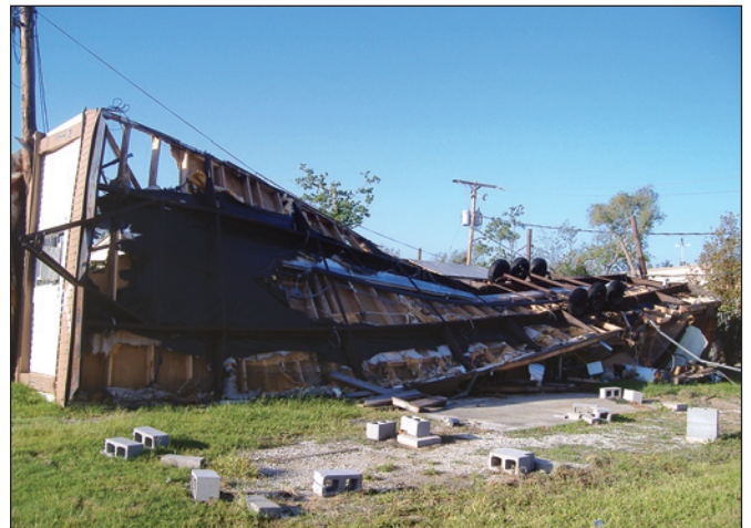
Figure 2-14. Manufactured home rolled over by Hurricane Katrina’s winds (Chalmette, Louisiana)
