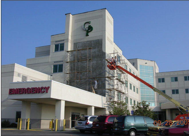
Figure 3-5. General view of Garden Park Medical Center. EIFS repairs were underway at the time the photograph was taken. The entire fourth floor nursing unit was taken off-line for about 1 month due to water leaks caused by roof membrane blow-off (Gulfport, Mississippi).
