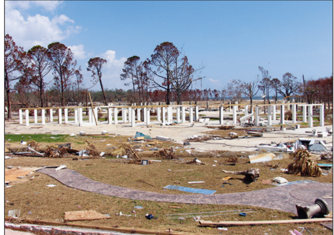
Figure 2-3. Typical building failures when surge and waves exceeded pier foundation height (Long Beach, Mississippi)
