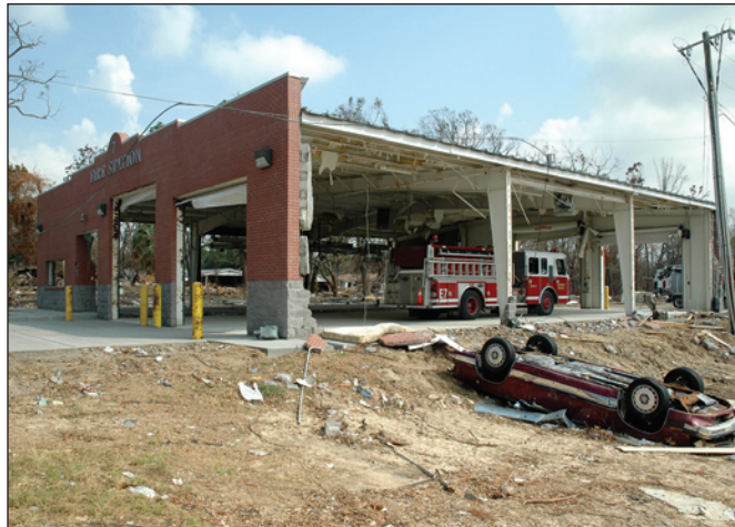
Figure 3-2. Newly constructed Gulfport Fire Station 7 destroyed by waves and storm surge (Gulfport, Mississippi)
