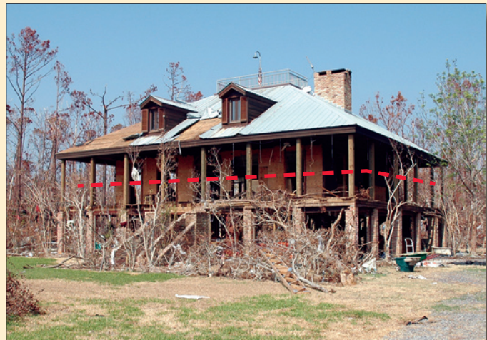
Wave damage to floors and walls, but pole construction left a repairable, surviving building.
