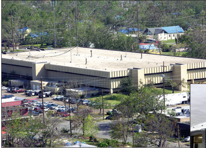
Figure 3-1. The EOC is located near the center of the first floor of the First Judicial District Courthouse in Gulfport. The windows and glazed doors were retrofitted with roll-down shutters, but communications tower damage and vehicle damage from roof aggregate still occurred (Gulfport, Mississippi).
