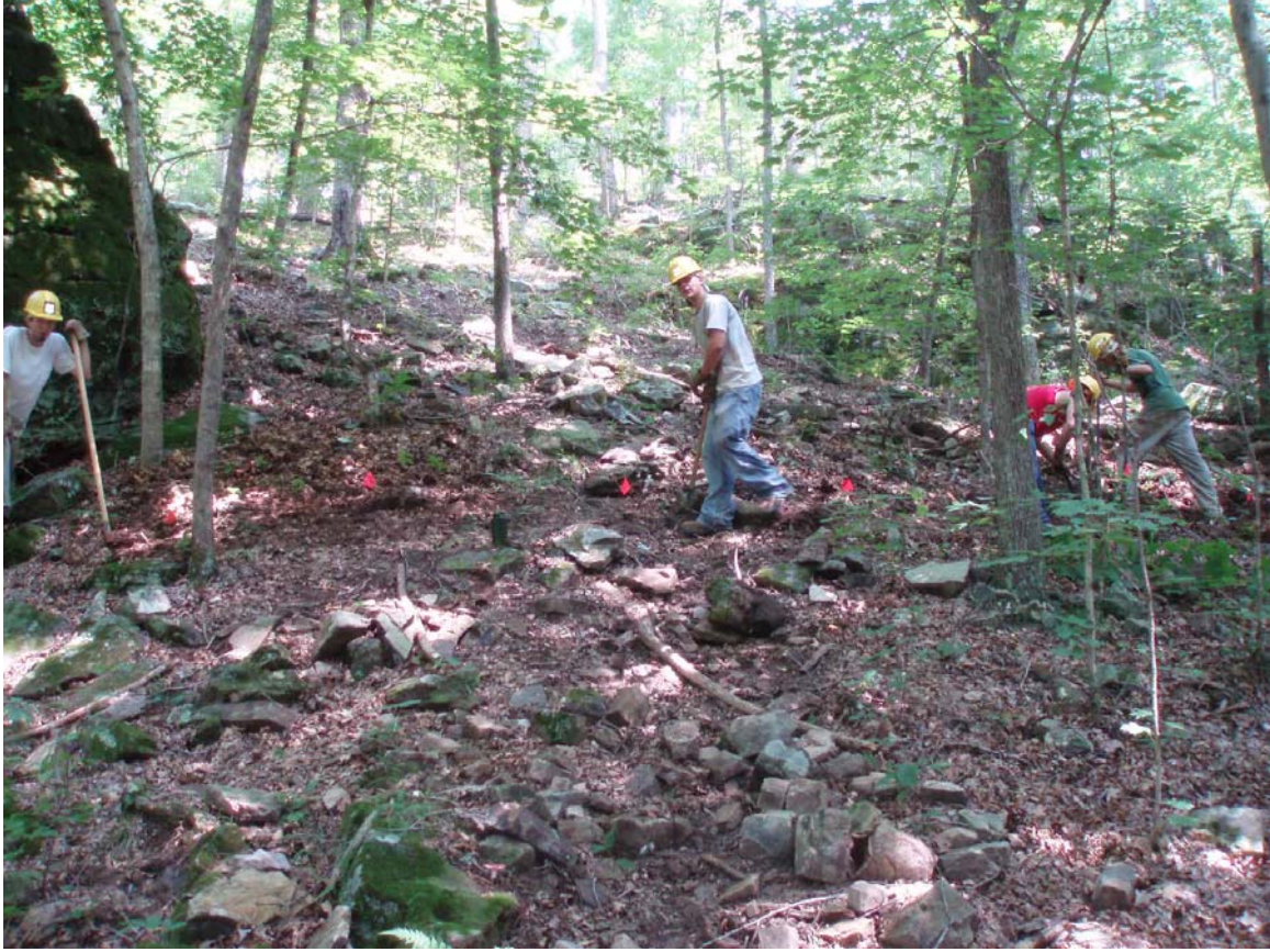
During construction. (Figure 2)
