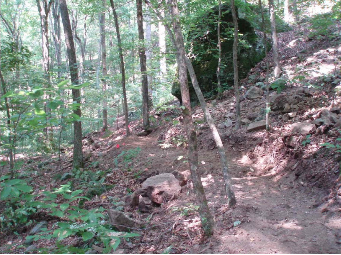
Almost done. Full bench cut, no-cut/fill. (Figure 4)
