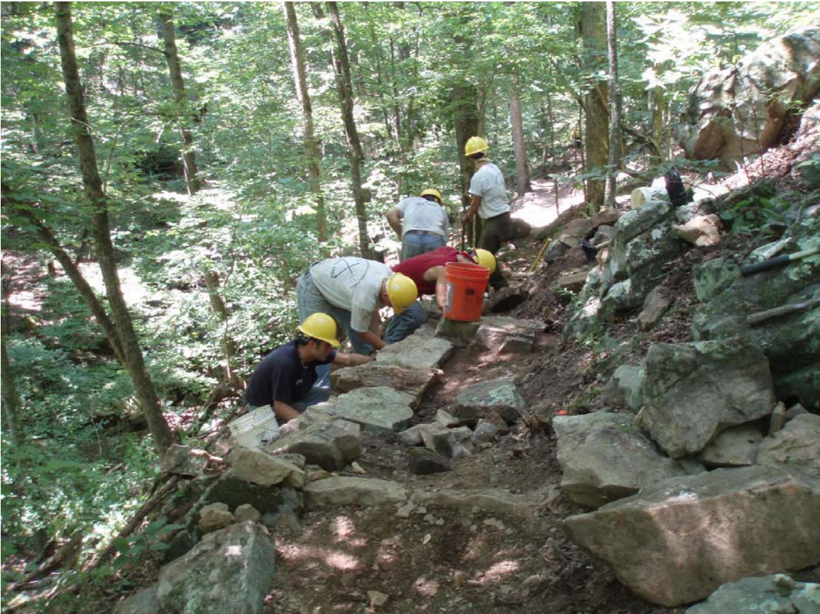
Side hill construction – rock steps and cribbing.
