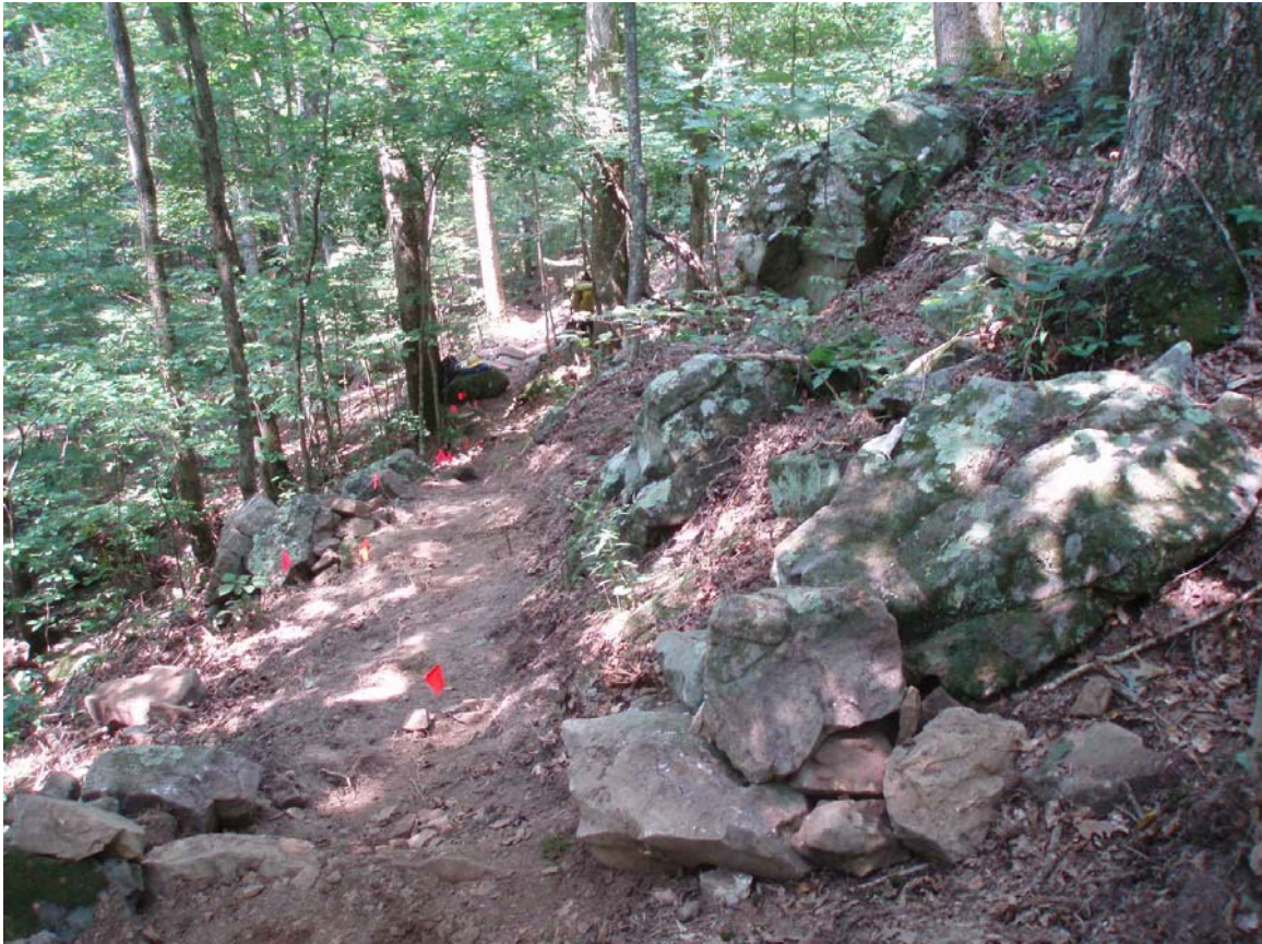
Side hill construction – early phase
