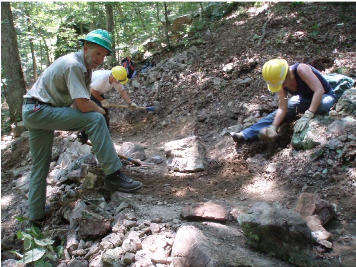
Finish tread work with rock cribbing.
