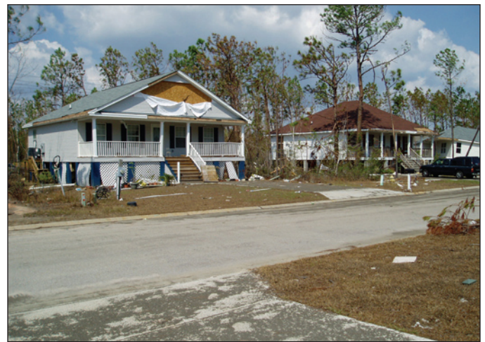
Figure 10. Although the site on the left is mapped Zone AE, proximity to the Gulf of Mexico shoreline and limited obstructions to waves indicate the site could be classified as a Coastal A Zone. The site on the right is over 4,000 feet from the Gulf shoreline and over 1,000 feet from the bayou, mapped as Zone AE, and has a base flood stillwater level sufficient to support >1.5-foot wave heights – but obstructions to waves (e.g., trees and other buildings between the site and the shoreline), and distance from the sources of flooding would indicate the area is not a Coastal A Zone.
