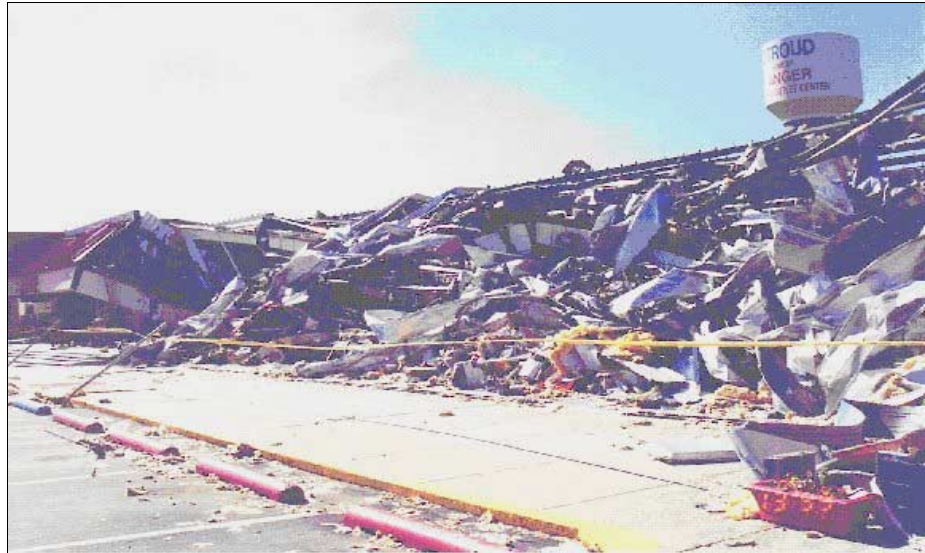
FIGURE 5-9: Stroud Regional Outlet Mall, Stroud, Oklahoma was struck by the vortex of a moderate tornado.
