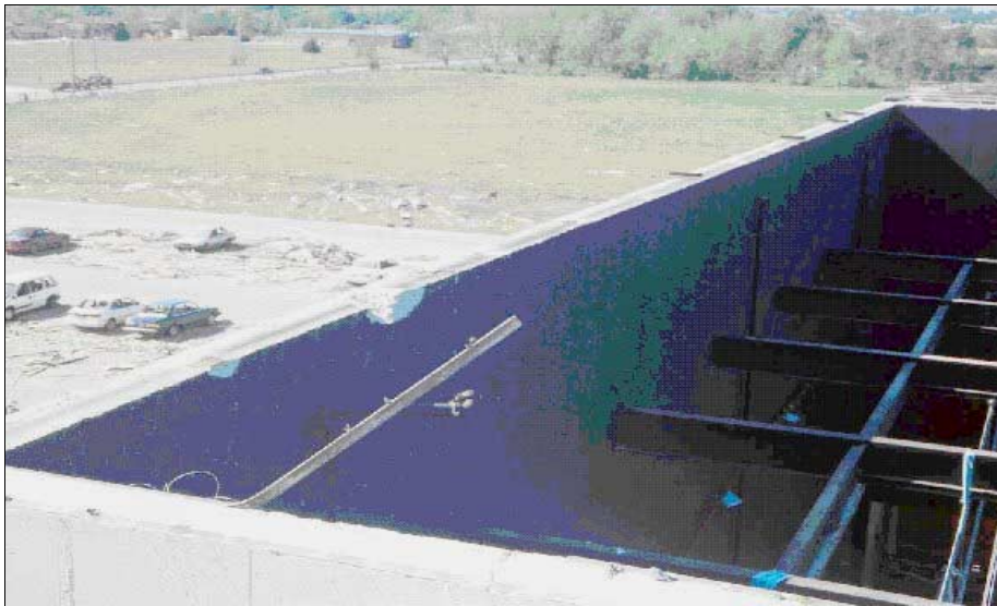
FIGURE 5-14: Roof blown off over top of auditorium at Westmoore High School, Moore, Oklahoma hit by inflow winds of violent tornado.
