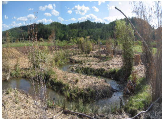
After the project, the stream grade, meander, and riparian vegetation were restored.
