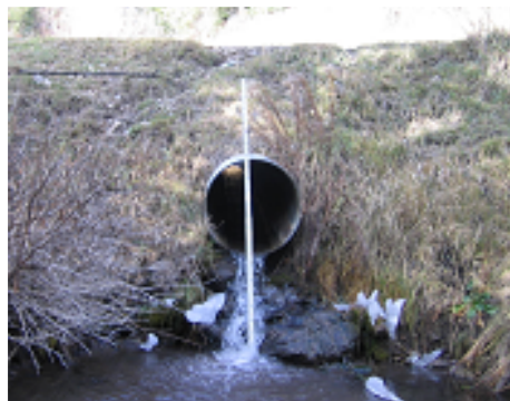
Horseshoe Creek culvert before replacement.
