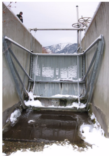
Georgetown Irrigation District Hydro headgate to be bypassed in 2009.
