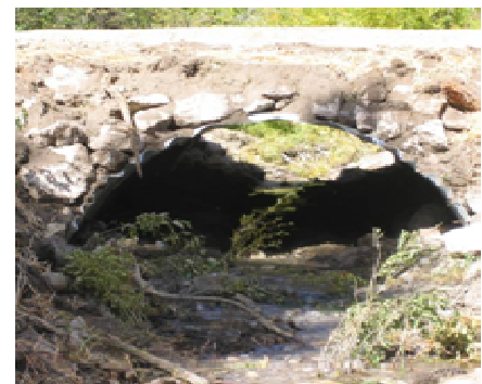
Crossing after culvert replacement.
