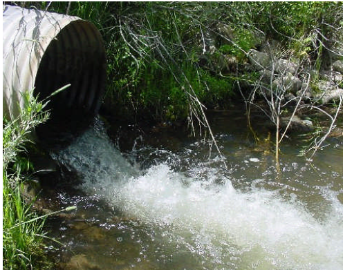
Burns Creek culvert outlet under McCoy Creek Road prior to replacement (2005).
