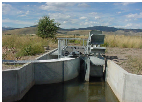
The fish screen and bypass at the Taylor Diversion constructed in 2004 and 2005.
