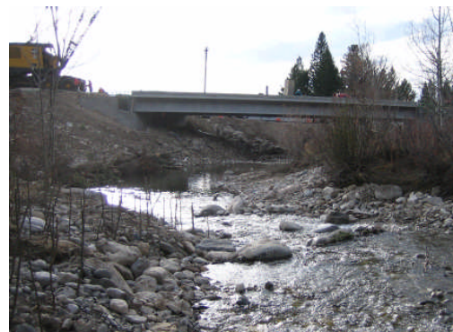
The Targhee Creek crossing at Highway 20 in 2005. The impassable culvert has been replaced by a fish-friendly bridge.
