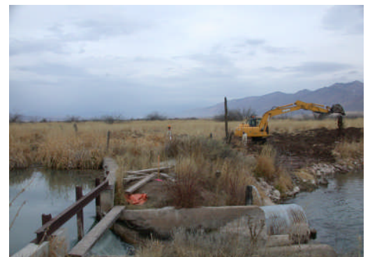
A bypass channel is excavated around the Peterson Diversion during fall 2005.
