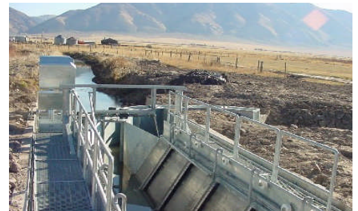
Newly constructed Fish screen and bypass channel at the Thomas Fork Diversion.
