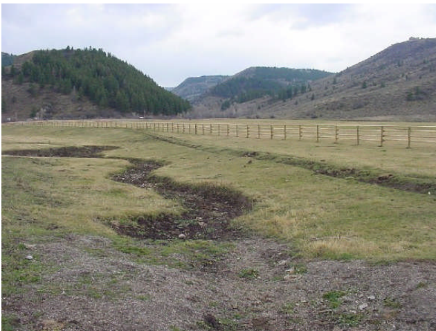
The newly excavated channel for Garden Creek meanders through Conant Valley Ranch between the Forest and the South Fork. A newly installed 4-pole fence protects the stream from livestock.
