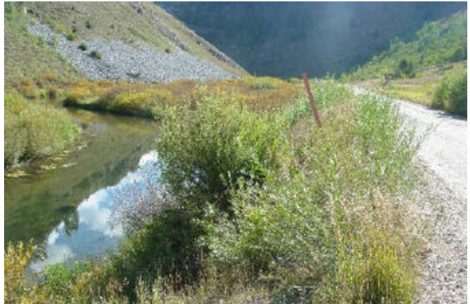
The Blackfoot River Road in the Narrows encroaches upon the Blackfoot River, important habitat for Yellowstone cutthroat trout. The Caribou-Targhee National Forest, in cooperation with Caribou County, hardened the road to decrease sediment delivery to the river.
