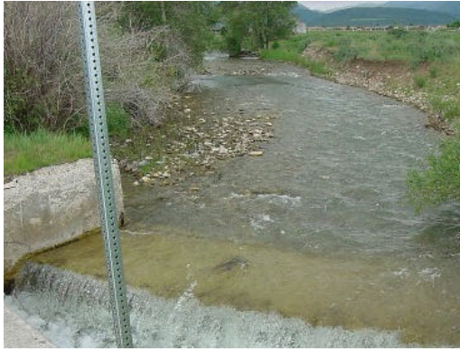
Before the project, an irrigation sill and concrete approach blocked fish passage from the Teton River and lower Trail Creek to quality fish habitat on the Forest.
