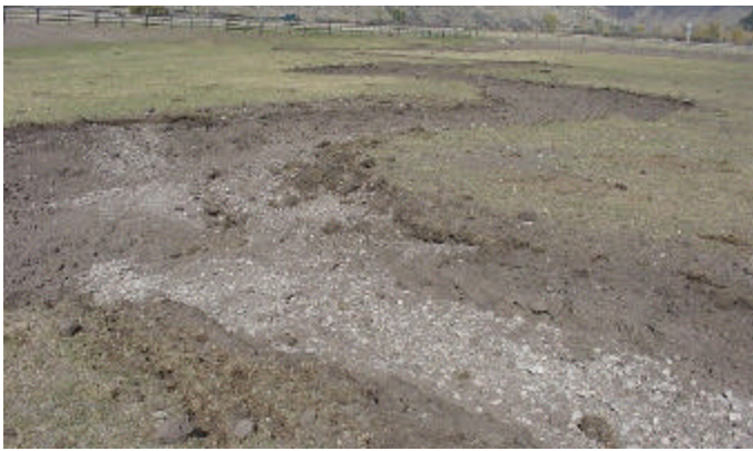
The newly excavated channel for Garden Creek meanders through Conant Valley Ranch between the South Fork and the Forest. Note gravels from old stream channel were uncovered
