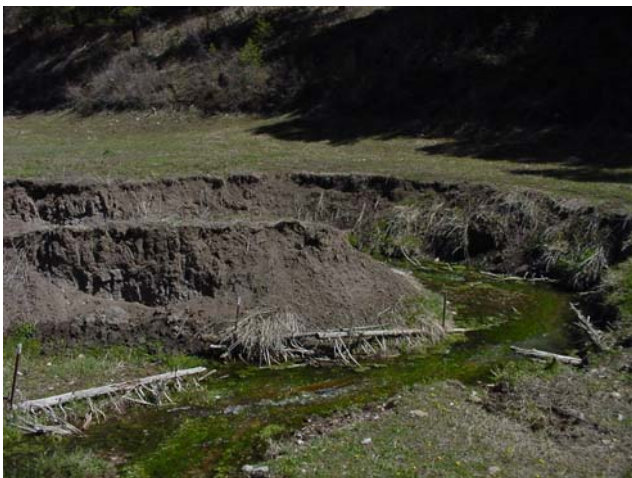
The raw, eroding stream banks of Pritchard Creek as it flows through the bed of the old reservoir. The project proposes to excavate these stream banks back at a slope and plant native vegetation to decrease erosion and increase stream shade.
