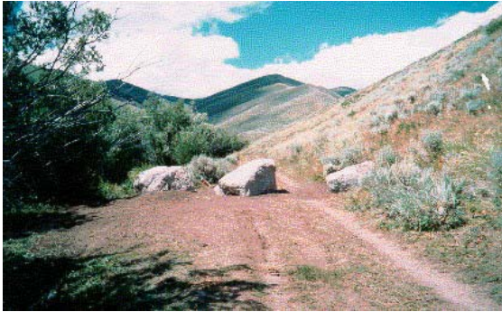
Strategically placed boulders physically convert a streamside road to a trail along the West Fork of Indian Ck, Dubois RD.
