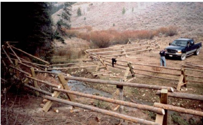
In Fall 2001, a fence was constructed along Preuss Creek, a major Bonneville cutthroat trout stream, to exclude cattle using the livestock driveway.
