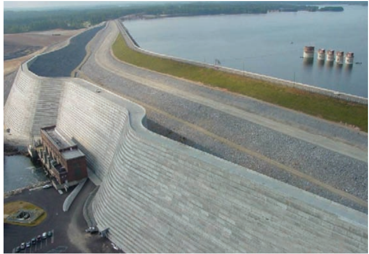
Saluda Dam reconstruction.
