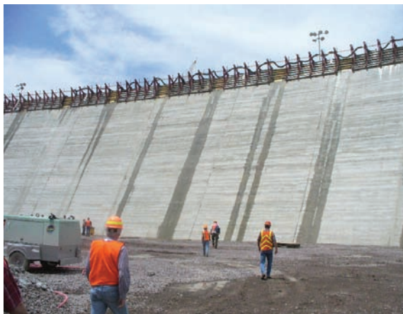
Inspection of Taum Sauk Project.
