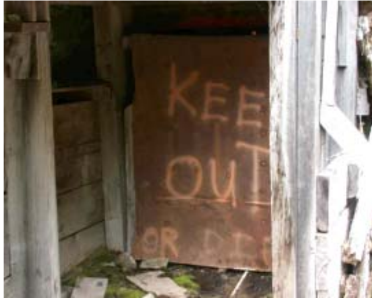
Photo 5. Level 4: Main Adit (photo by D. Boles)
