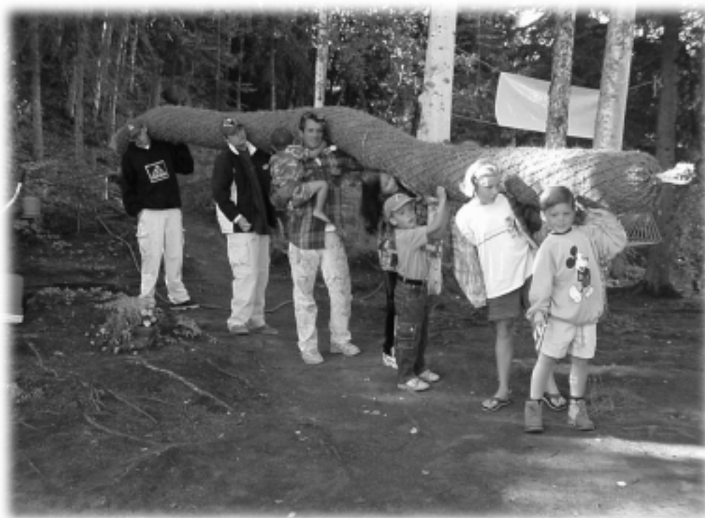
Restoration is a family affair! Sherman family members carry a fiber "log" that will be used to help stabilize the shoreline.
