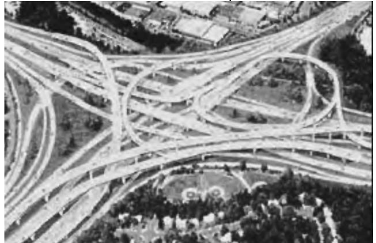
Figure 1-1. Springfield, Virginia, interchange.
