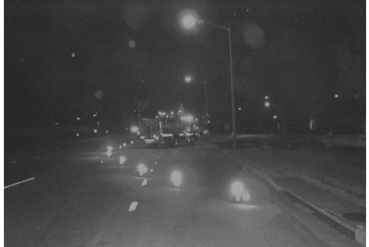
Figure 5-13. Flares are more visible than traffic cones during nighttime operations.
