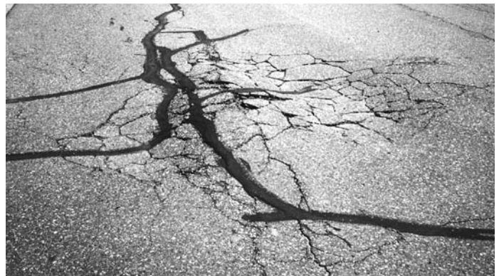
▲ Frost heave damage from spring break-up.
