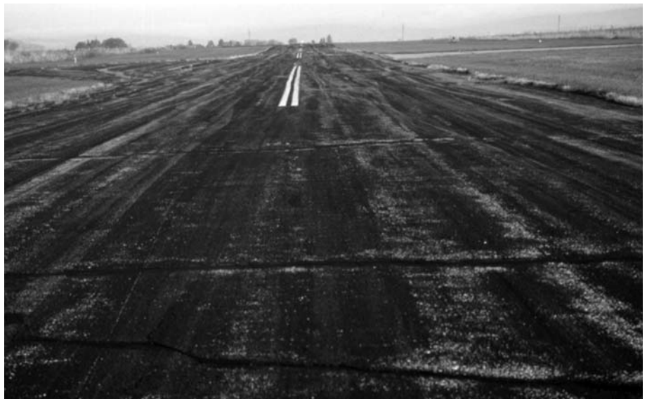
▼ Worn sealcoat needs new surface treatment.
