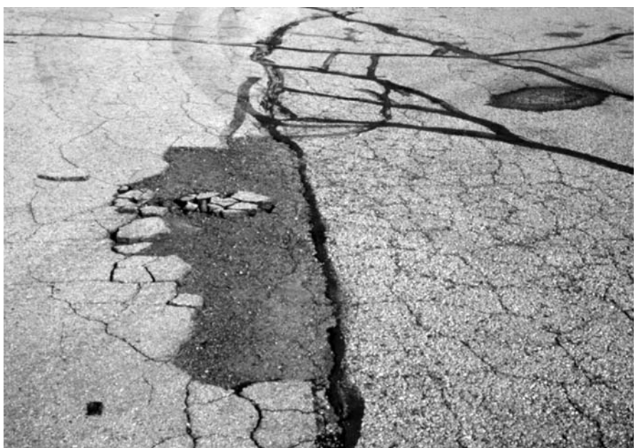
▶ Extensive failed pavement and debris.
