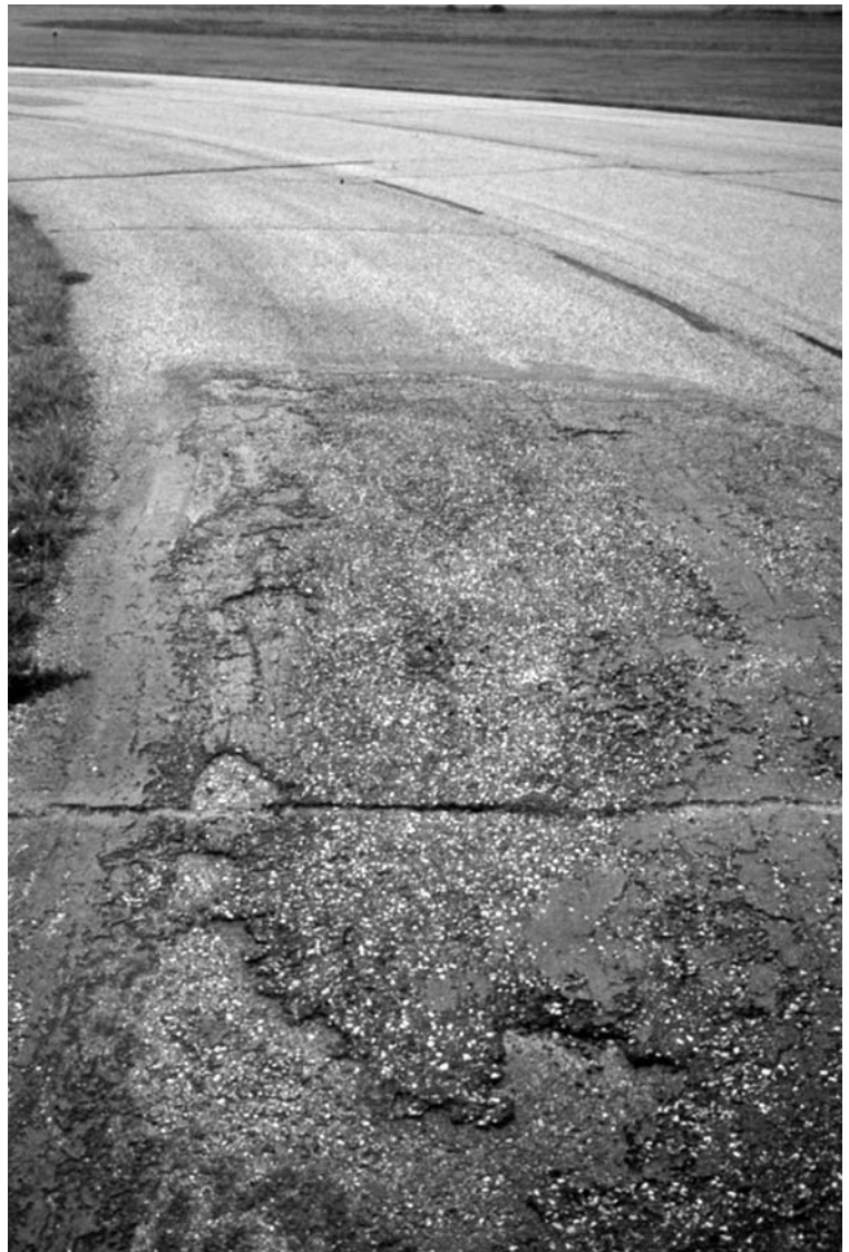
▶ Patched area in poor condition.
