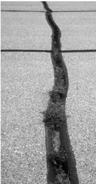
▲ Widely spaced, well-sealed cracks.
