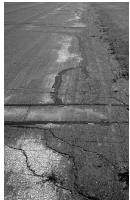
▼ Repair broken pavement and apply overlay.
