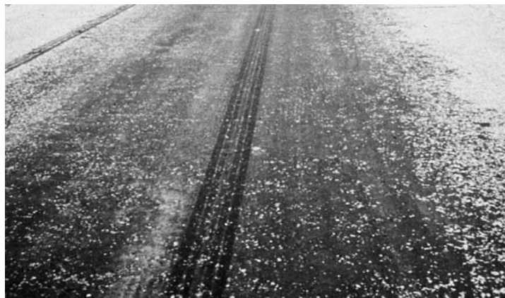
◀ Flushing. Dark patches show where asphalt has worked to surface.
