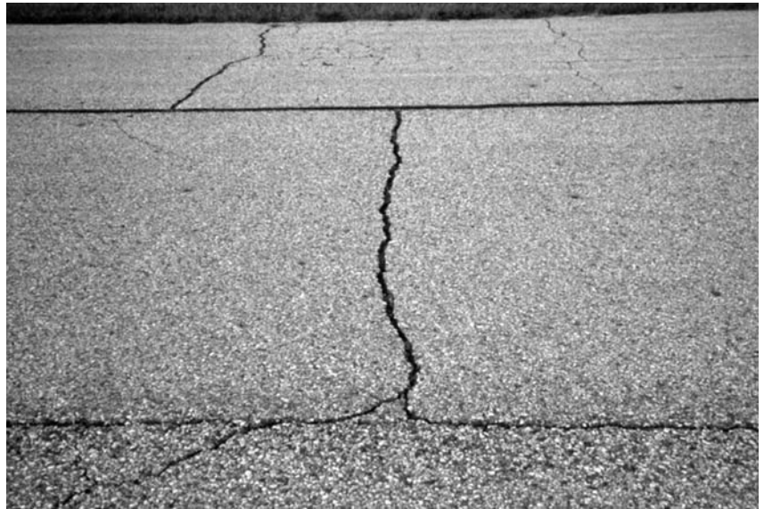
▶ Right angle cracking forms blocks.
