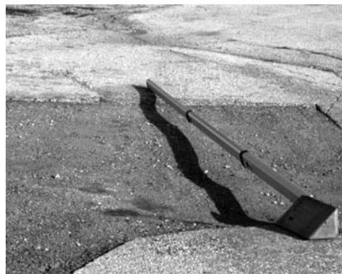
▲ Frost heave damage from spring break-up.
