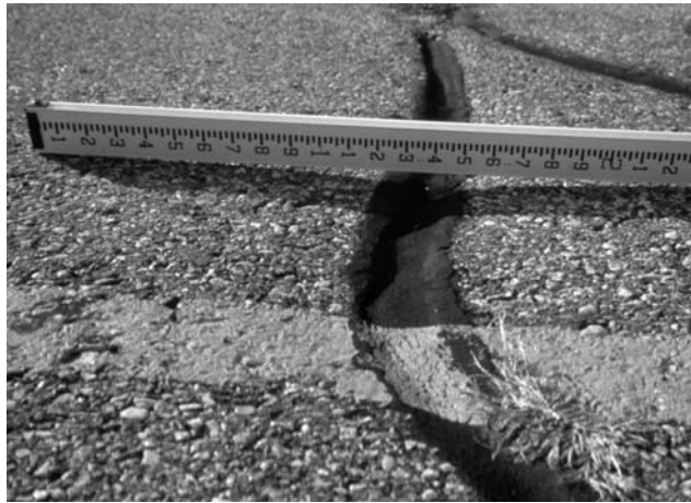
◀ Edge cracking at several locations.
