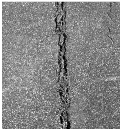
▲ Wide cracks with no sealant.
