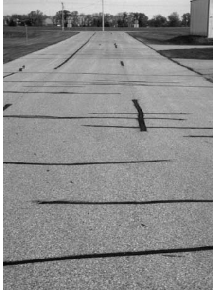
▲ Widely spaced, well-sealed cracks.
