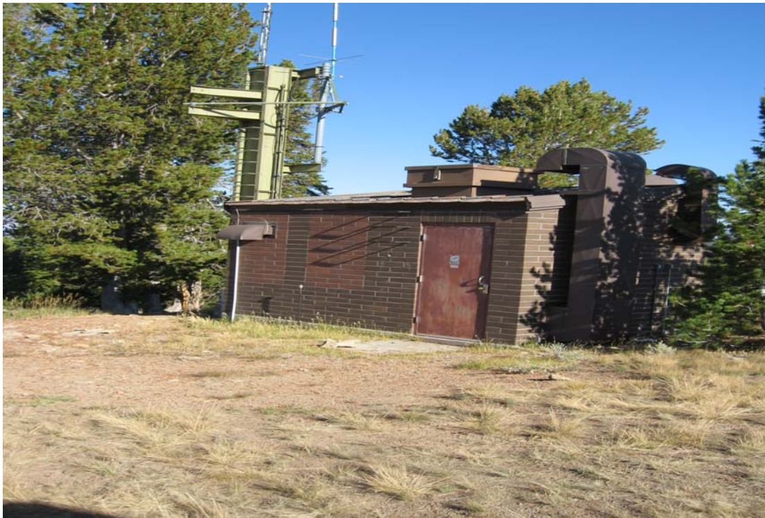
Photo 3: Existing Sawtooth Telephone Company communication facility on Galena.
