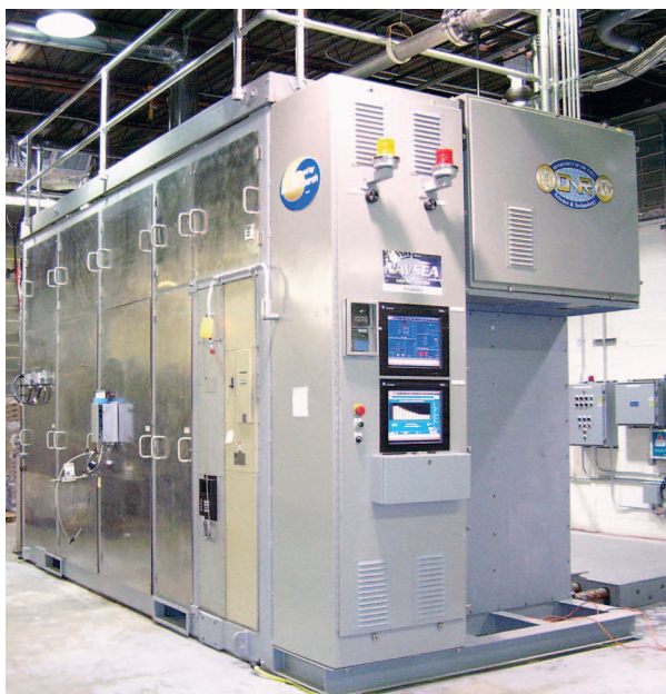
Hot box. The 625 Molten Carbonate Fuel Cell Reformer System (fuel cell stack is out of view) produces methane from high-sulfur logistics fuel to power the fuel cell stack with an expected efficiency of 47–50%. The system is being land-tested by the Office of Naval Research, and will be installed at the Naval Sea System Command's engineering facilities in Philadelphia in 2007 for extended testing.
