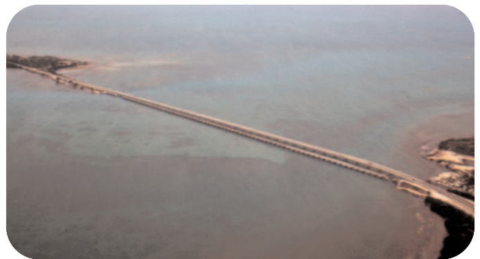
An aerial view of a portion of the seven-mile bridge shows the tidal cut between Vaca Key and Pigeon Key. Tidal waters flow through the cuts between the Keys, connecting the Atlantic Ocean and Florida Bay.
