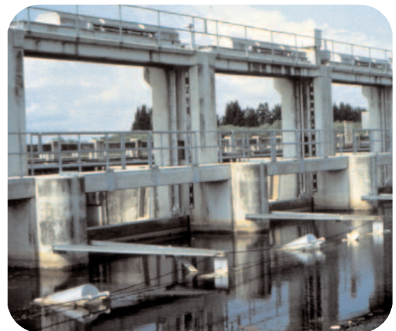
Canals, levees, and water control structures were built to control the flow of surface waters in South Florida. (Photo: William Nuttle)
