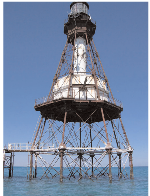
Fowey Rocks Lighthouse, located on the reefline off Miami, is one of the reef lighthouses that houses SEAKEYS oceanographic and meteorological instruments. The reef lighthouses, built along the reef tract in the 1800s, are navigational aids maintained by the U.S. Coast Guard. Photo: SEAKEYS
