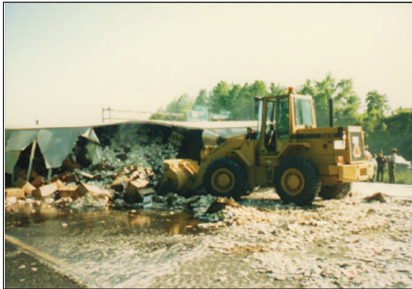
Figure 3-12: Clearance of a tractor-trailer accident
