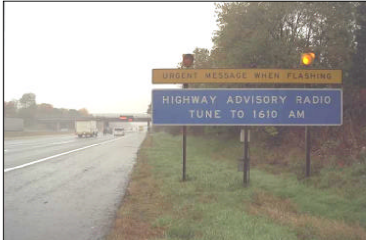
Figure 3-3: HAR station with warning lights
