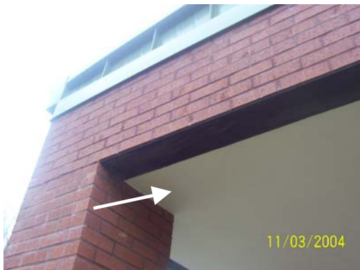
Figure 11. Drywall applied as outdoor porch ceiling
