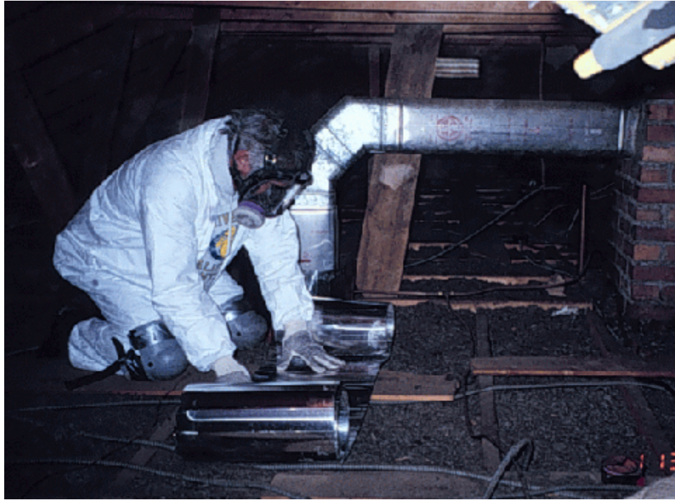
Appendix F – Picture 1. Preparation of attic for future CI application.
