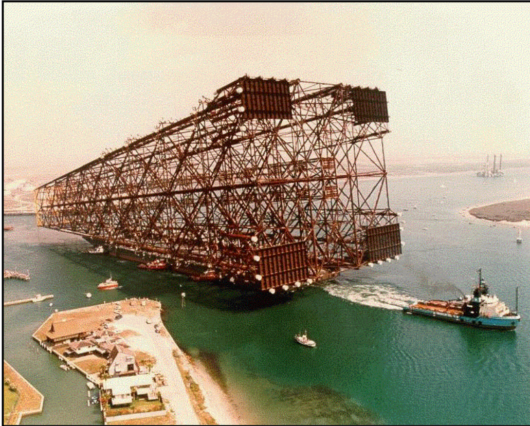
Figure 2.1: Bullwinkle steel jacket leaving Corpus Christi. Courtesy of Shell Deepwater Development Systems Inc.
