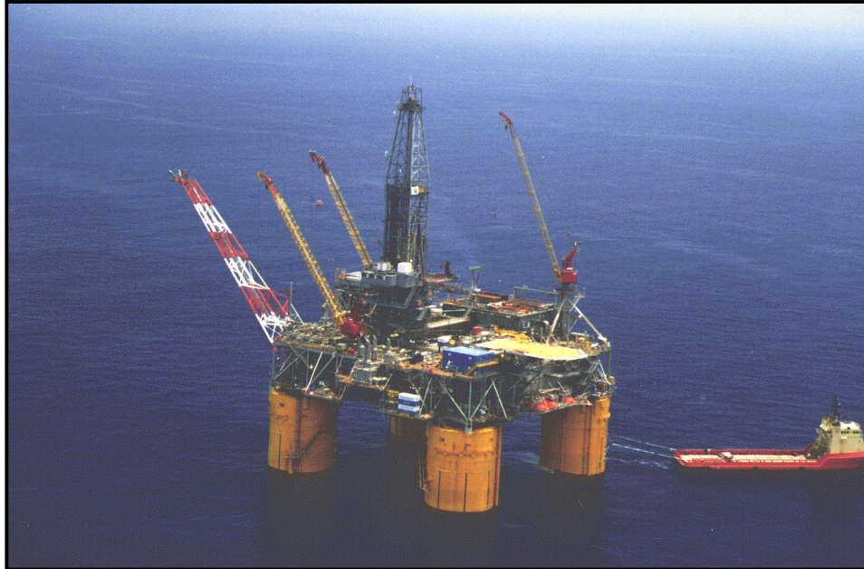
Figure 5.5: Mars TLP being towed to the Mississippi Canyon location. Courtesy of Shell Offshore Inc.
