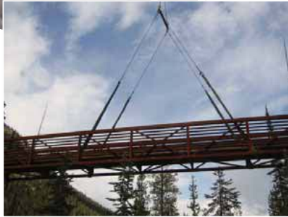
Photos: Bridge installation on Heather Lake trail
