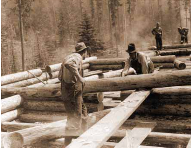
CCC workers building the Salmon Meadows Lodge
