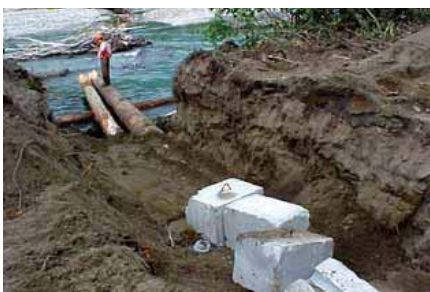
Photo above shows completed logjam project. Photo at right shows same view before project—the road completely washed away. Photo below of logs being placed and anchored in old roadbed.
