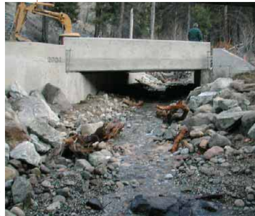
The photo above is the new bridge over Stormy Creek.
