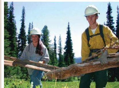
Maintenance on Bear Creek Trail, Naches Ranger District
