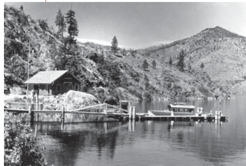
25-Mile Guard Station and boat dock
