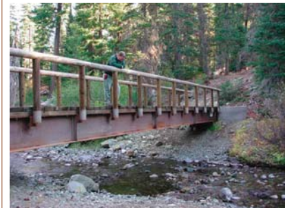
New bridge at Deroux Creek, Cle Elum Ranger District
