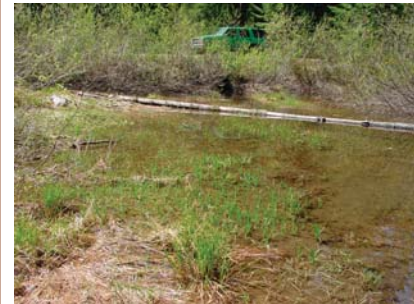
Before. One of three oxbow channels disconnected from the White River by road fill and an undersized culvert (dark spot below green vehicle).
