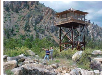
Columbia Breaks Fire Interpretive Center
