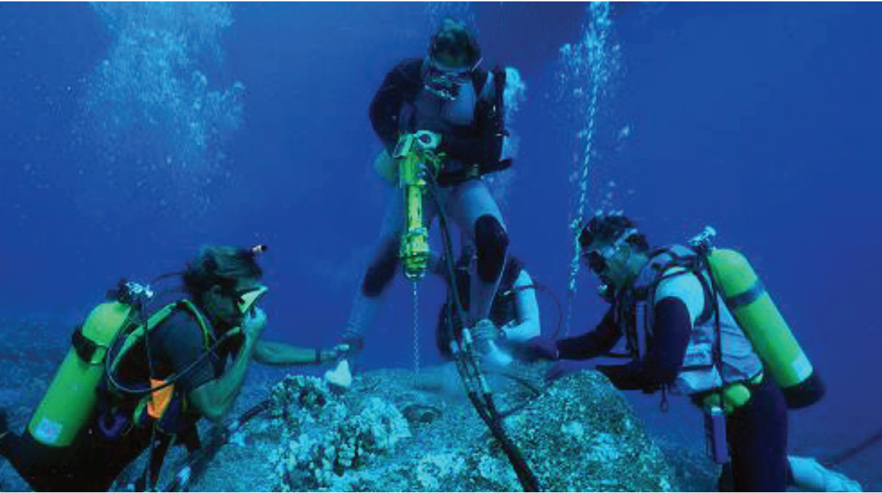
Divers prepare substrate for placement of mooring buoys.
