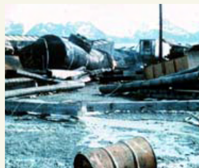
Tsunami damage at Seward, Alaska, following 1964 Good Friday Earthquake. (Photo: NOAA)
