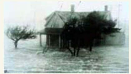
Storm surge swamps a house. (Photo: NOAA)
