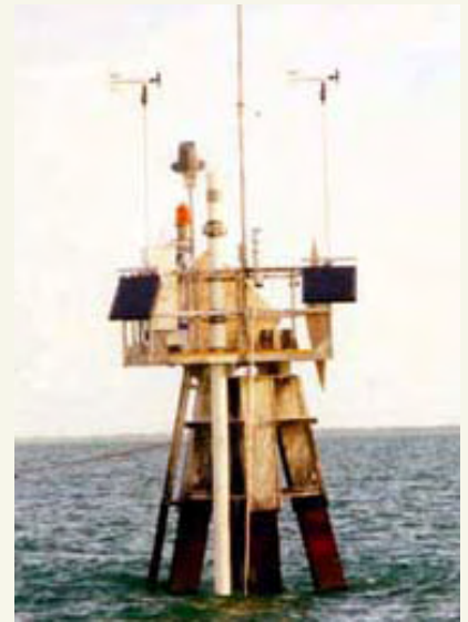
Seakeys stations transmit real-time data. (Photo: NOAA)
