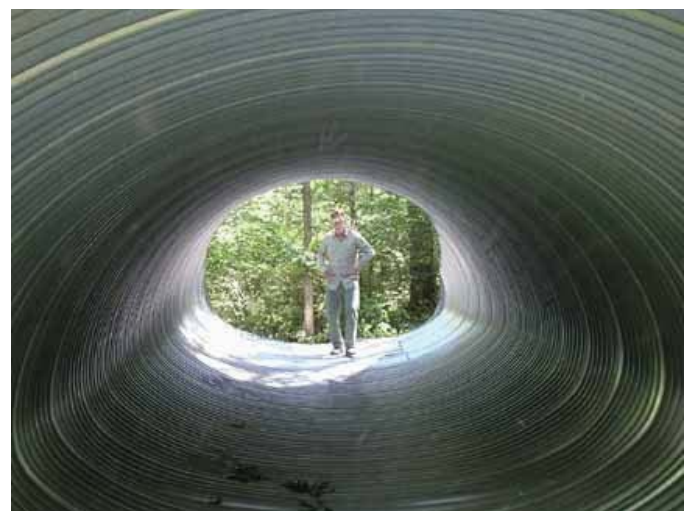
New culverts allow aquatic critters to easily pass under road/stream crossings.
