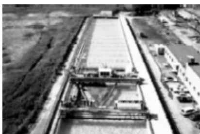
Figure 33: Ohmsett facility in New Jersey.
