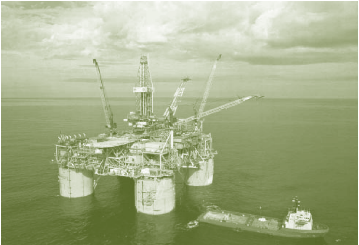
Shell's "Ursa" tension leg platform in the Gulf of Mexico.
