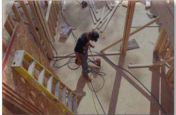
Figure 2. Reducing the risk of back injury and fatigue using a simple extension for a light nail gun.
