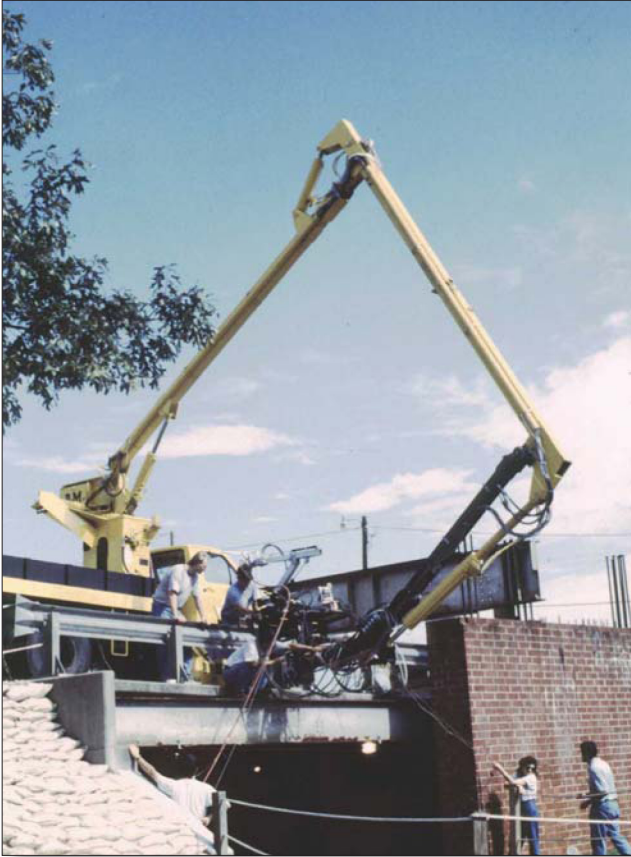
Figure 4. The RBPR containment performing the robotic CO 2 blasting.
