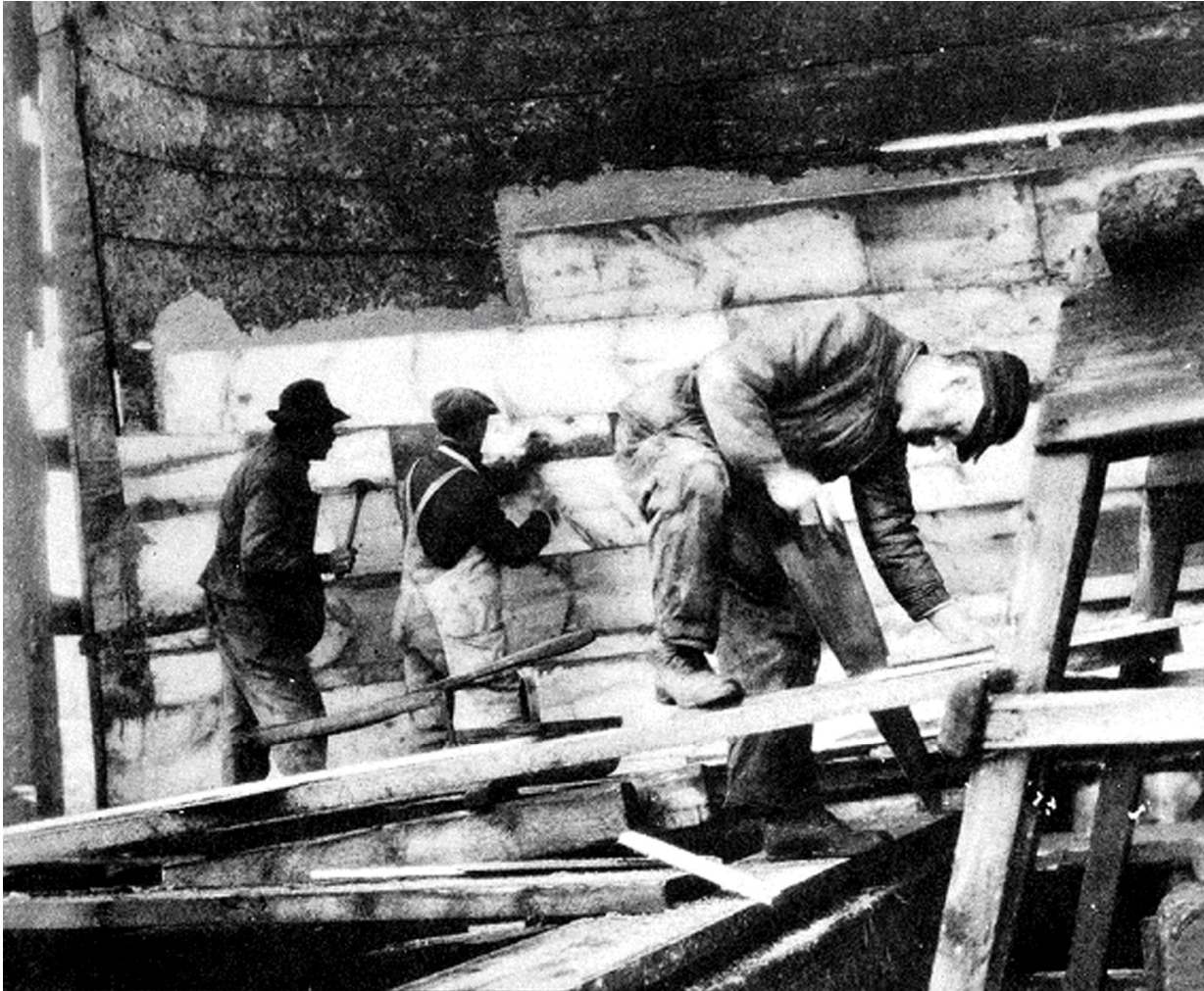
Figure A2. Carpenters applying pine sheathing before the application of metallic sheathing (From Church 1938, Figure 17).
