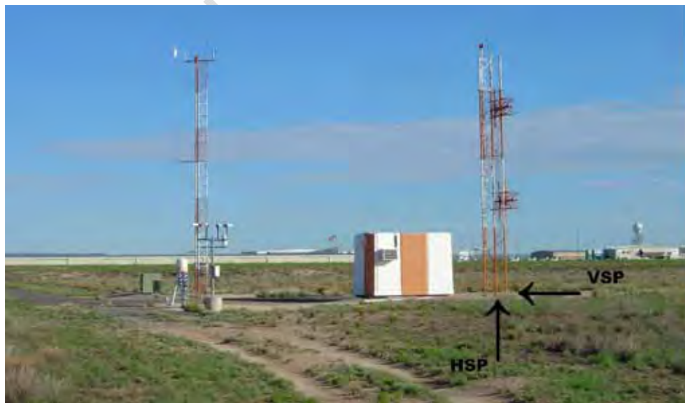
Figure C-6. Typical glideslope installation.
