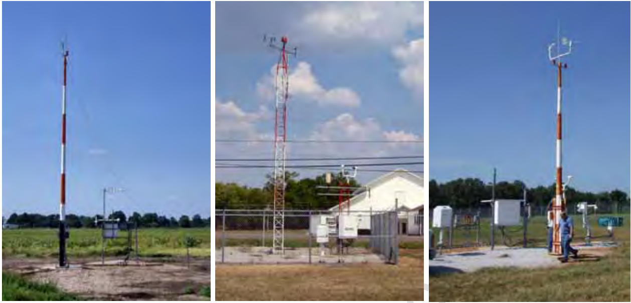
Figure 2-10. SAWS, AWOS and ASOS Station Installations.
