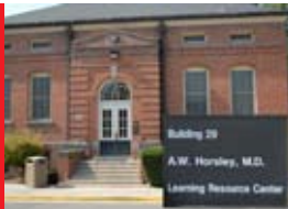
Building 29, Boise VA
