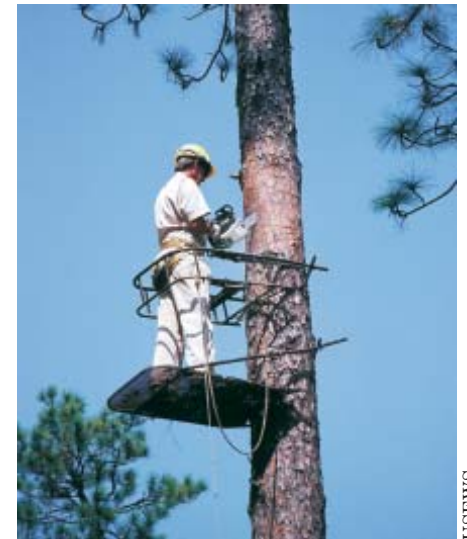
Installing artificial RCW cavity
