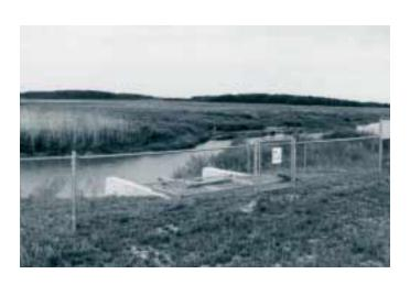
Freshwater Impoundments Tour Stop 3 The ability to manipulate water levels in these pools is the key to creating necessary habitats. Pool levels are maintained by the use of water control structures with stoplogs. In the spring, excess water in the pool is released to the salt marsh to create mudflats which provide a food source for wading birds and shorebirds.
