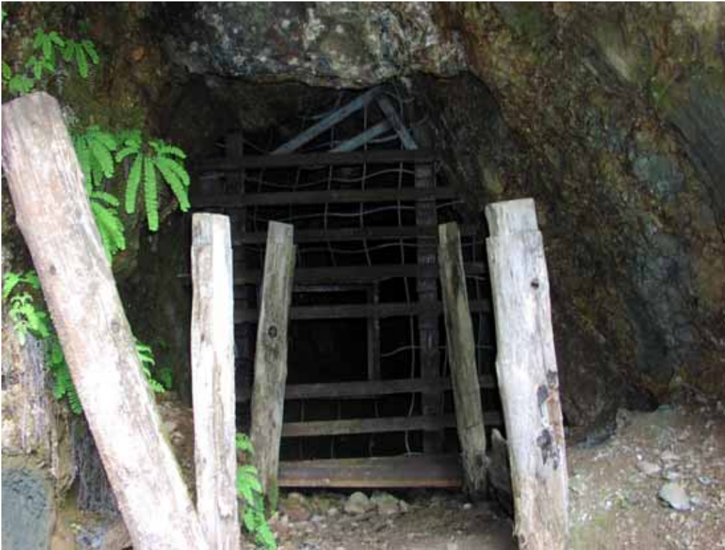
Photograph 18. Closeup of Adit 1 at the Kiggins Mine
