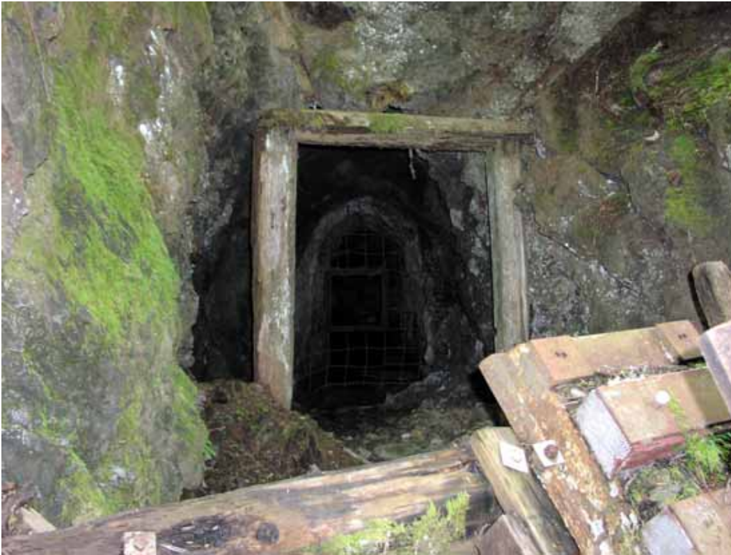
Photograph 26. View of Adit 1 at the Nisbet Mine
