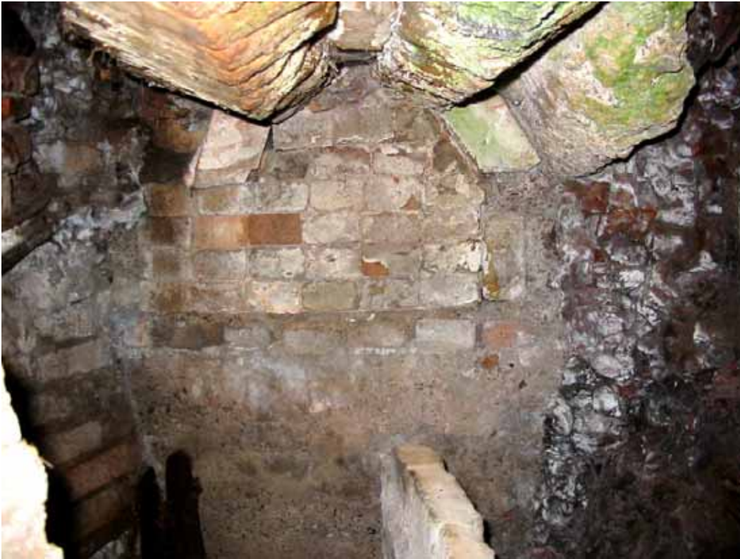
Photograph 14. View inside Kiggins Mine Furnace
