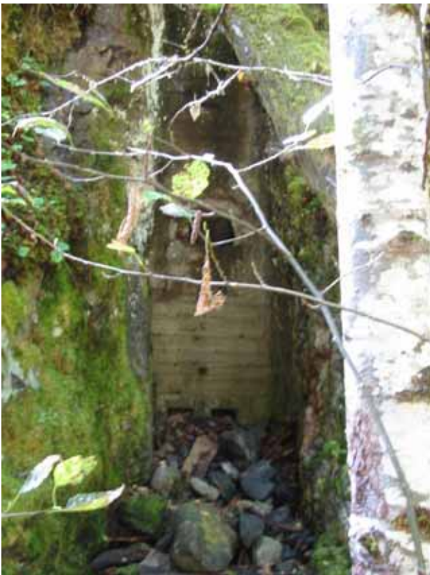
Photograph 15. View of the Kiggins Mine Furnace, above the Oak Grove Fork
