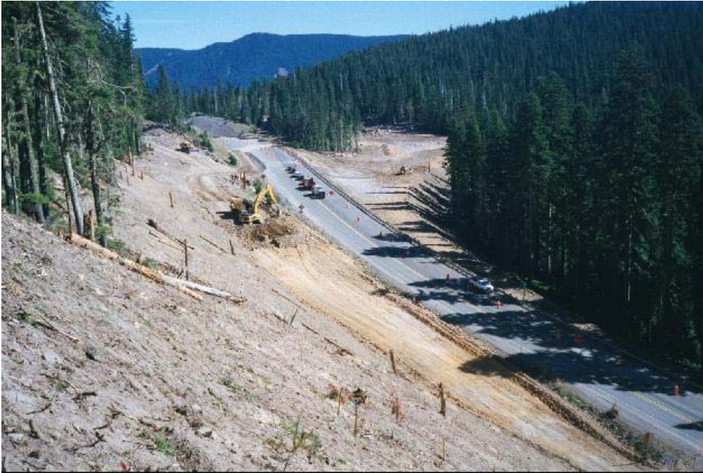
Hwy 35 slope during construction, 1999
