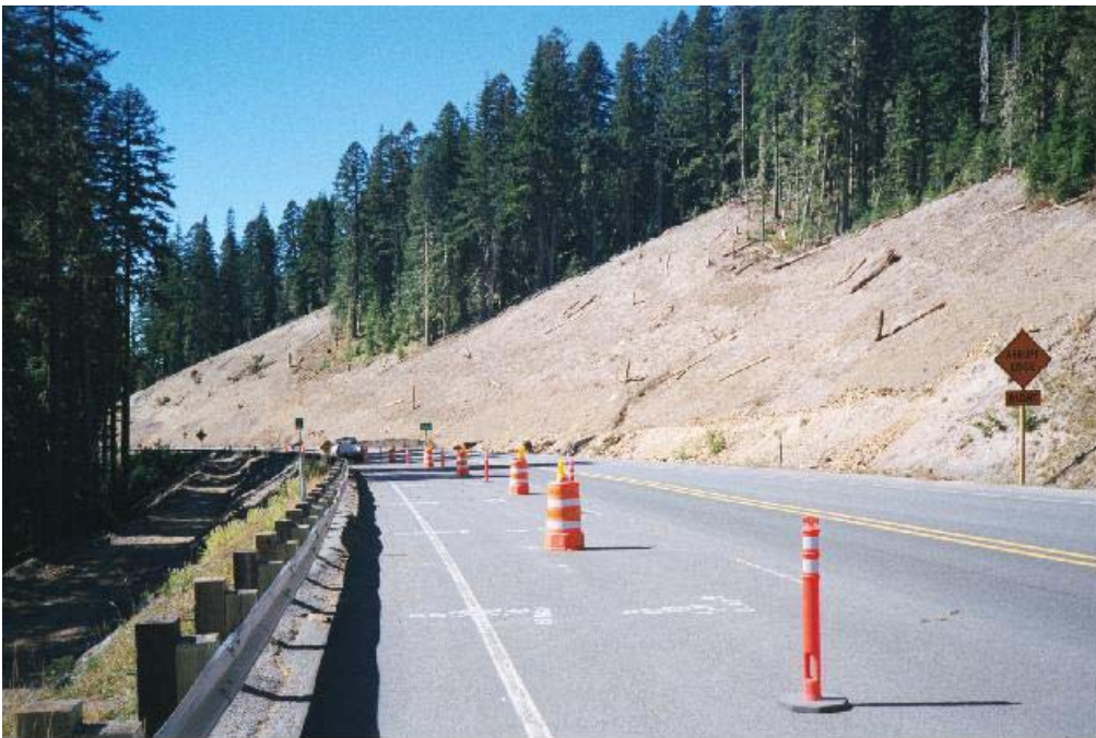
Hwy 35 Slope Before Hydroseeding, 1999 Slope Was Treated October 1999
