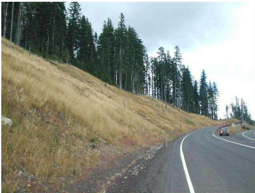
Hwy 35 Slope, August 2001 Very Good Native Plant Establishment
