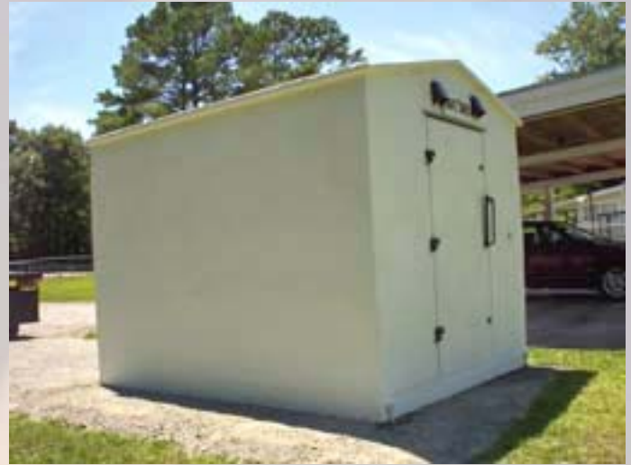
Figure 5-5. An example of a tornado "safe room" for either exterior or interior home use.
