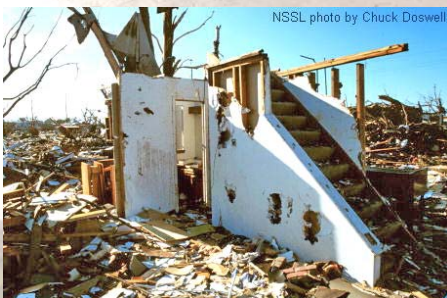
Figure 5-9. Stairwell among debris.
