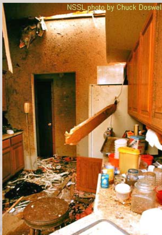
Figure 5-3. An example of tornado debris that has been turned into a flying projectile.
