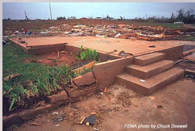
Figure 5-2. This is classic F5 damage. The Bridge Creek/Moore, Oklahoma, tornado of 3 May 1999 leveled this house, swept the foundation almost completely clean, shredded the house remains into small pieces and scattered the debris downwind to the northeast (rear). The house was relatively well-constructed with slab-to-wall anchor bolts evenly spaced around the bottom plate. Some of those bolts can be seen in this photo, protruding upward from just inside the edges of the concrete slab.
