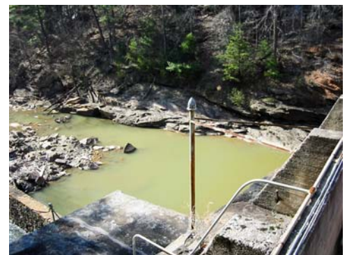
Woodside II Dam scheduled to be removed to restore free-flowing Twelvemile Creek. Both photos credit Industrial Economics Inc.
